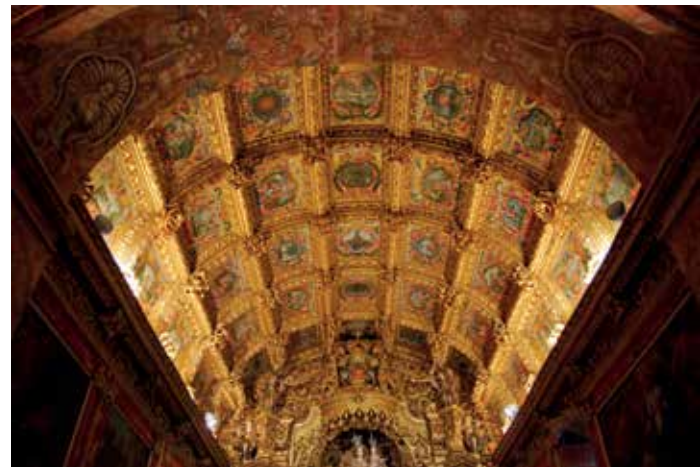
17 Wooden coffered ceiling with applied emblematics, second third of 18 th c., Chapel of Our Lady of Hope, Abrunhosa, Portugal
